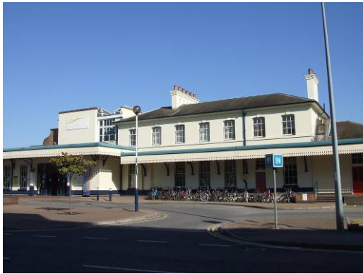
Eastleigh Railway Station – lots of bike racking and well presented.
